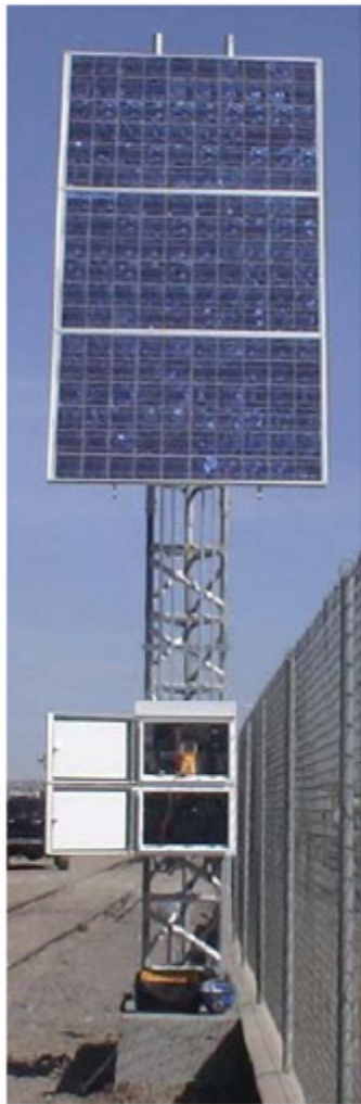
20 Foot tower with solar
